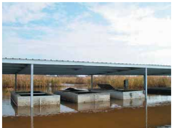
Figure 3. Flooded alligator tanks.
