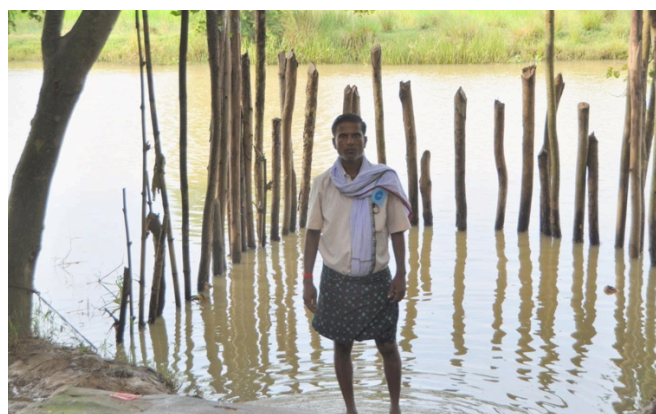
Figure 6. Balaram Patra stands where he experienced a non-fatal attack in June 2010, at Ostia village. The forest department constructed this ‘safety barrier’, which has worked as a deterrent, but is not a secure system as there are many gaps and missing timber through which a crocodile can pass.
