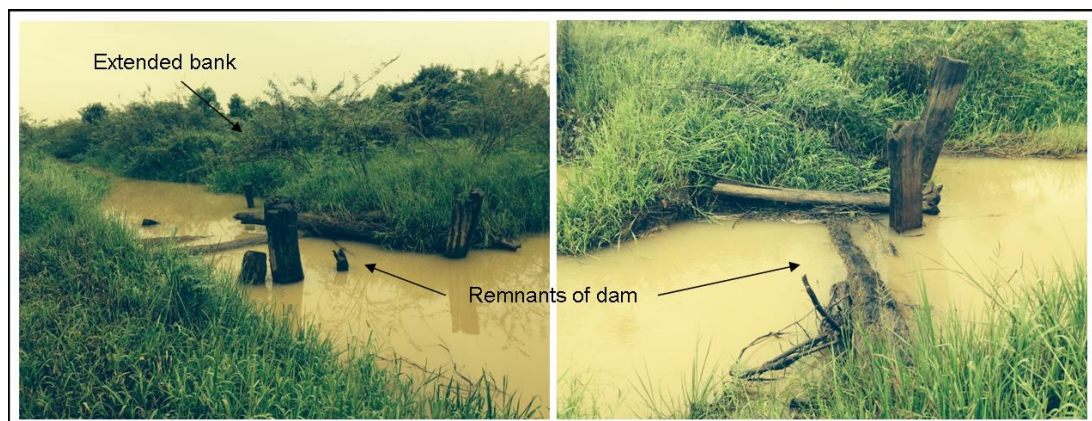
Figure 5. Tributary that flows in from the east to Lake Mesangat. Remnants of a dam washed away during recent flooding. The northern bank had reportedly been extended and built up, which effectively constricted flow into Mesangat.
