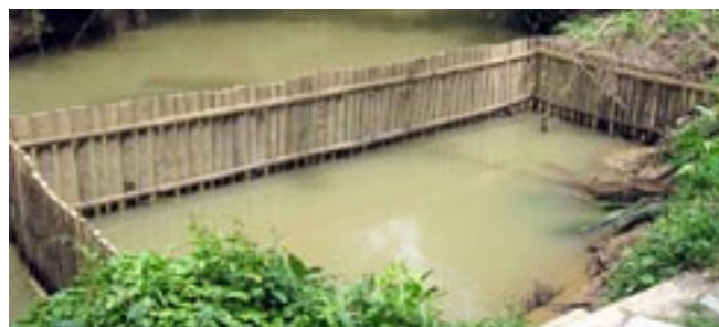
Figure 3. Crocodile exclusion enclosures and fences typically have three sides fenced, and are open to the bank. Photograph: Anslem de Silva.
