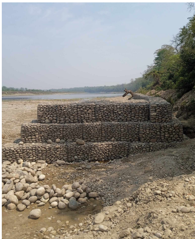
Figure 2. Newly constructed gabion wall along bank of the Rapti River in CNP. Photograph: Bed Khadka.
